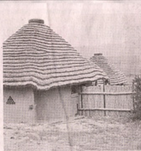
A visitors' centre at Qwa Qwa looking on to the Maluti Mountains is inspired by indigenous principles and construction
